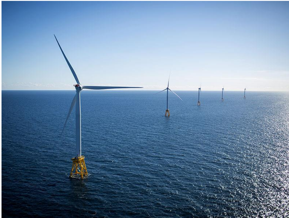
Fig. 1: Saudi Aramco and General Electric announce joint wind turbine venture
